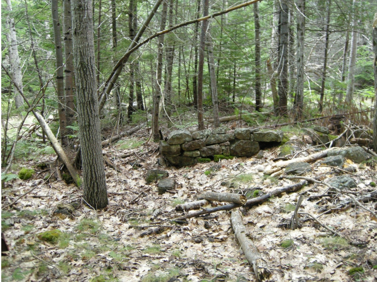
Photograph believed to be foundation of Second Pest House at Eagle Lake. 8/4/2010
