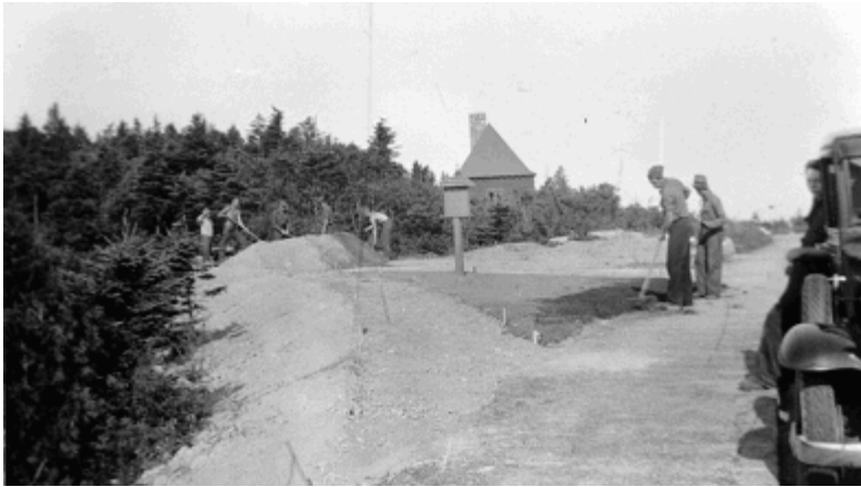
Figure 15. View looking west at CCC crews dressing a new trail to the Cadillac Tavern, c.1934. The Ranger Station in the background. It now serves as the trailhead of the Cadillac Mountain South Ridge Trail. (RM-147, 347_1, Acadia NP Archives)
