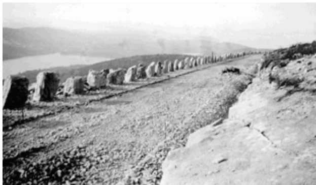
Figure 7. View of Cadillac Mountain Road below the current Blue Hill overlook, at Station 144, looking north to Station 140, ready for the application of asphalt. September 26, 1930. (Leo Grossman Personal Collection, #51-5.)
