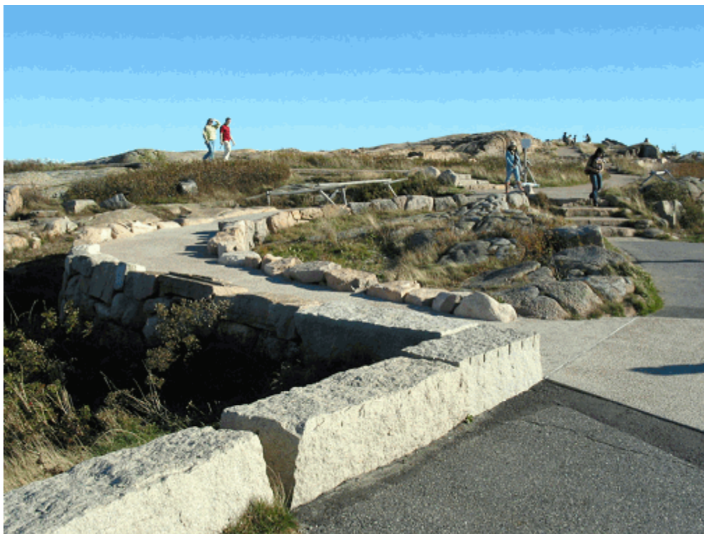
Figure 25. Accessibility on the Cadillac Summit Loop Trail was improved recently with construction of ramps. (OCLP 2007)
