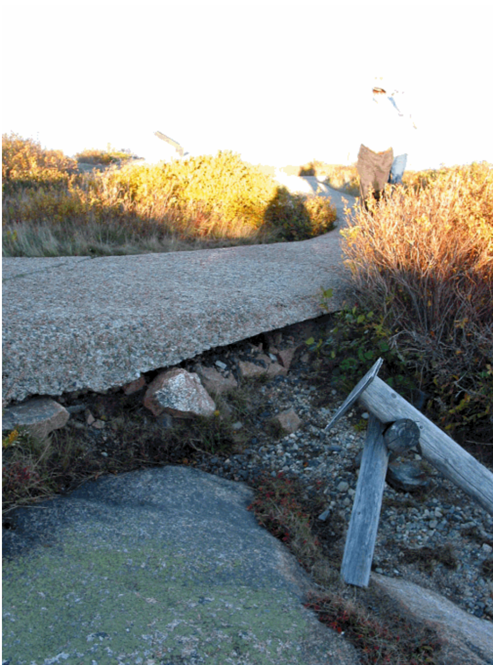
Figure 26. Erosion alongside the Cadillac Summit Loop Trail and development of social paths are major problems at the summit that threaten both visitor safety and sensitive vegetation. (OCLP 2007)
