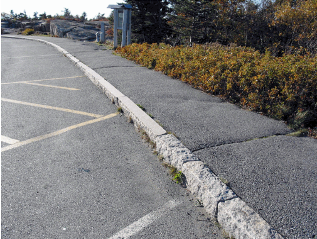
Figure 24. The character of the gray saw-cut granite curbs contrasts with the pink rough-cut granite curbs. (OCLP 2007)
