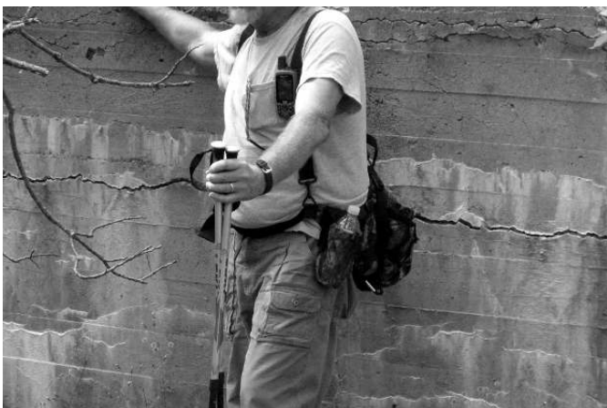
Cellar hole & foundation. Garage foundation at Rowell estate McFarland Mountain & Young · 20 Aug 2009
