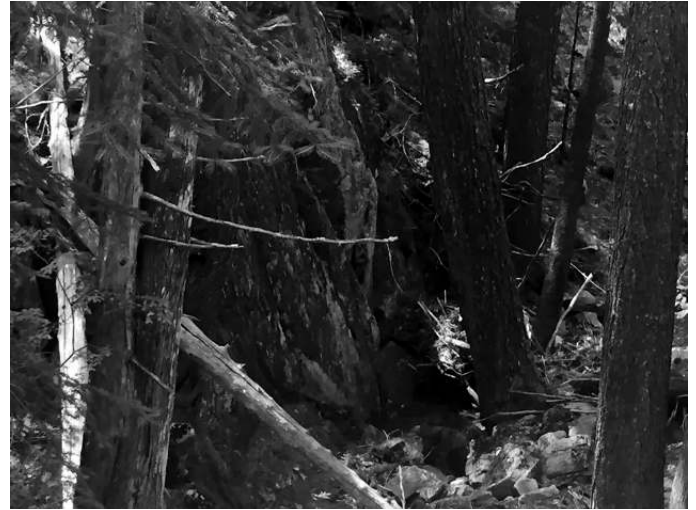
Top edge of "Old Sargent Ravine" i was following washout as possible road and ended on top of Ravine looking down. FALLS AWAY to culvert with incredible stone work going under the current drive · 22 Jul 2019
