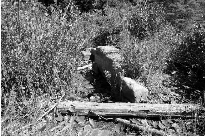
Bridge & abutment. Lake Wood. Granite Bridge over outlet. McFarland Mountain & Young · 24 Jul 2015
